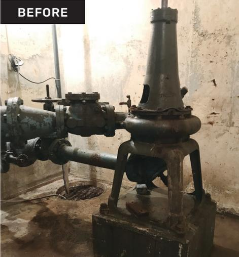
The existing shaft-driven centrifugal pumps, after nearly four decades in service.
