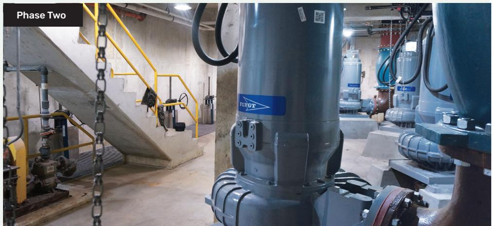
**PHASE TWO:** The City was so happy with their collection system upgrade that when the second phase of the Smart City initiative kicked off to replace their East Pump Station, the four specified pumps were Flygt Model CT-3356, 280 HP Dry Pit Submersible pumps. This design removed five floors of shafting and intermediate bearing supports, couplings, and guards. The pumps will never require specialty personnel for alignment and include a glycol closed
