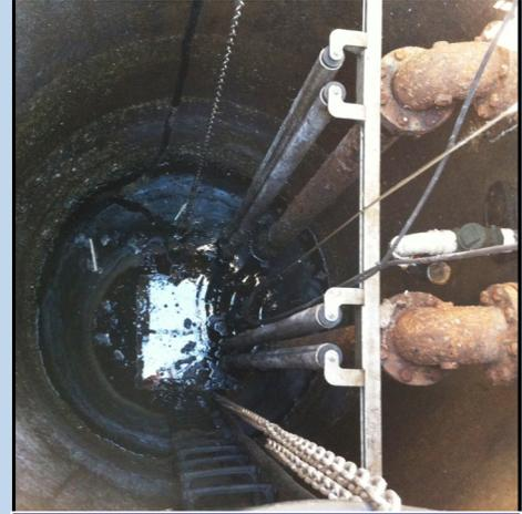
Flygt Pumps Easily Retrofitted onto the Existing Rails
