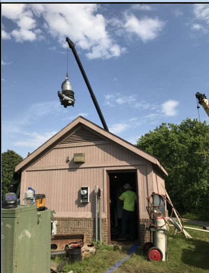
LOWERING NEW PUMP
