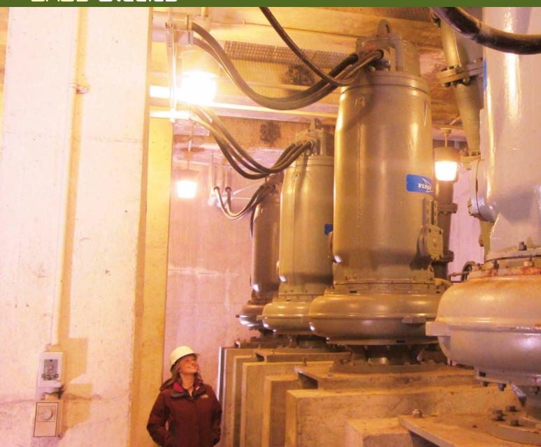
Flygt N pumps rated at 7.5 million gallons (28.4 million liters) per day each in flow capacity. Each pump has a VFD for flow control. Other improvements included replacement of the existing comminutor, all suction and discharge piping including valve and flow meter replacement, addition of a second redundant discharge header, yard piping, a standby power generator sized to run all four pumps, and related electrical and controls improvements.
