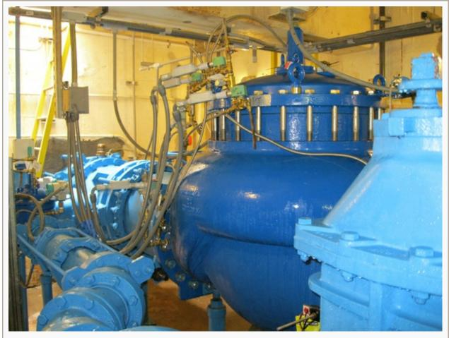
Pressure reducing valve provides remote SCADA control of flow and pressure. (Courtesy Singer Valve)
