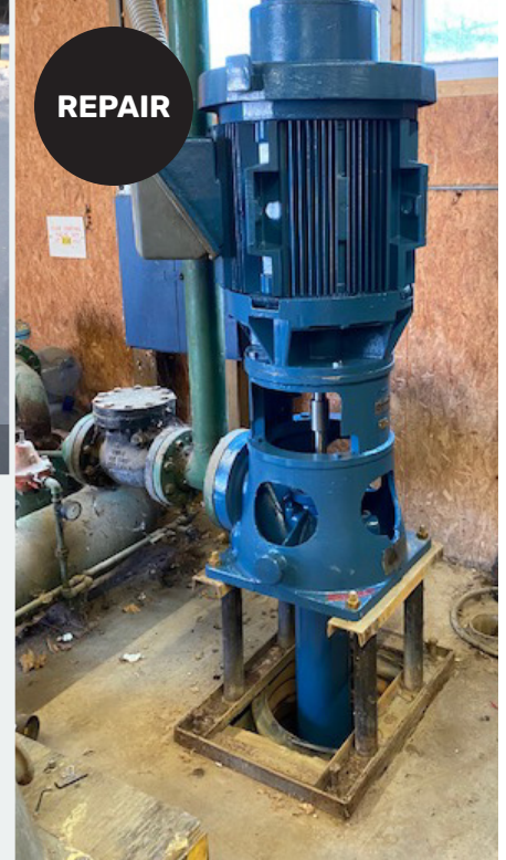
The rebuilt 8-stage vertical pump.
