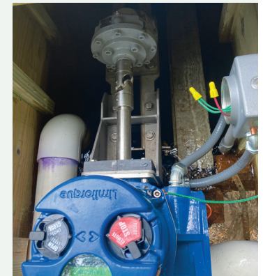
Limitorque electronic motor that operates Slide Gate 2 and controls flow coming into the mill.
