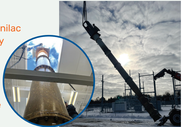
Re-installing pump with overhead crane.
